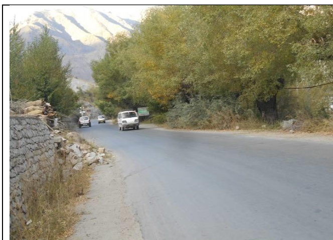
Fair Condition of Road at Km 1+800
